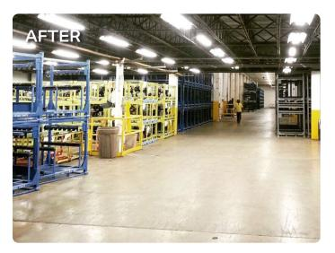
impacts to the operational budget were maximized. In addition, worker morale and energy improved with the correction of color temperature and color rendering. Overall, lighting energy use was reduced by more than 58%, while still achieving significant increases in illumination.
